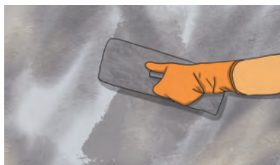
Figure 6.19: Applying plaster on the wall
