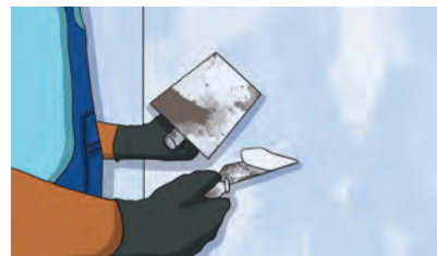
Figure 6.20: Plastering of a wall
