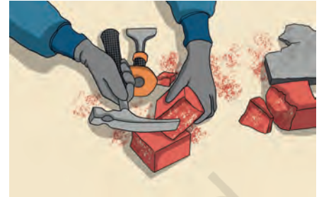
Figure 6.16: Cutting the brick using chisel and hammer
