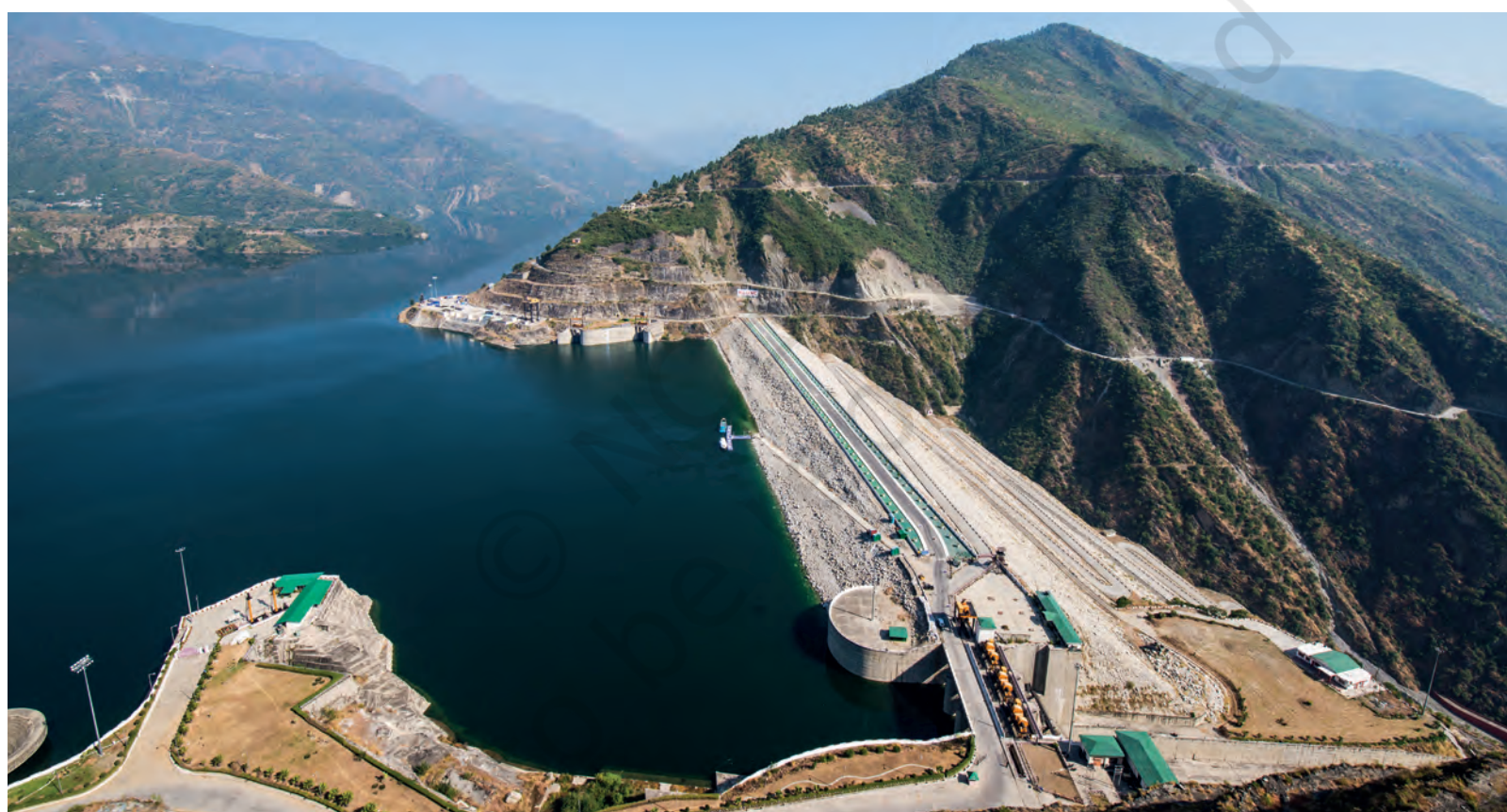
Figure 6.1: Tehri dam in Uttarakhand
